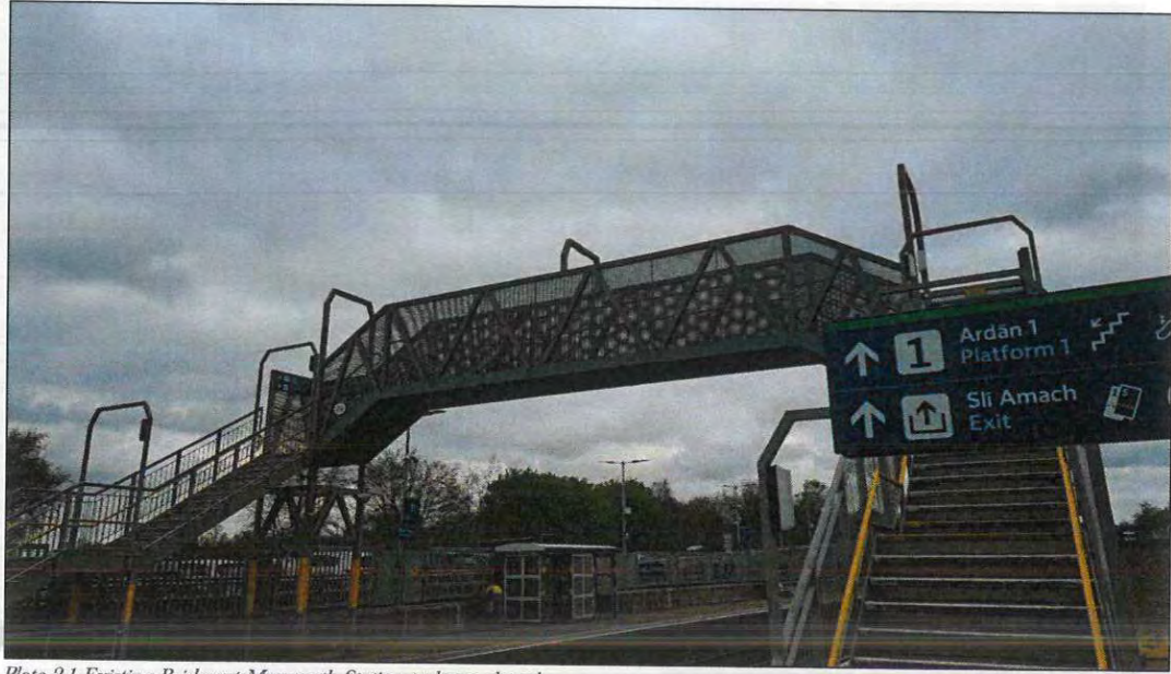
Plate 2-1 Existing Bridge at Maynooth Station to be replaced
