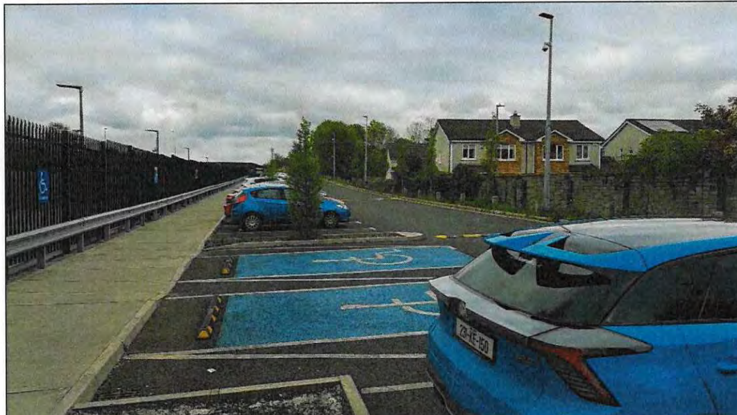
Plate 5-2 Car park to the South of the existing bridge where the main compound will be located
