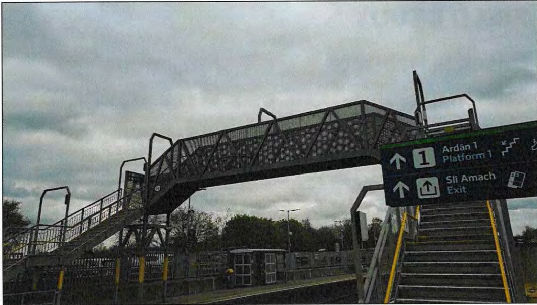
Plate 5-1 Existing Bridge at Maynooth Station to be replaced
